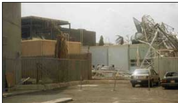
A bad situation made even worse: The telephone company's tower at their central office fell... directly onto the electricity transfer panel, rendering their emergency generator useless.
